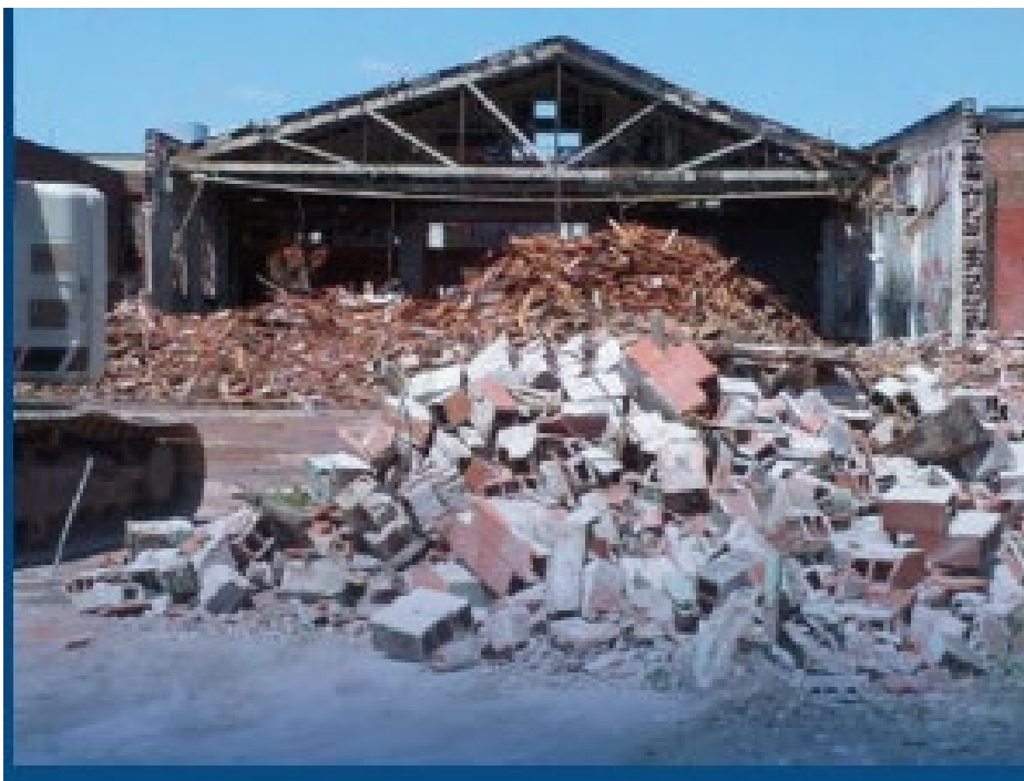
BEFORE: Auto Repair and Machine Shop
